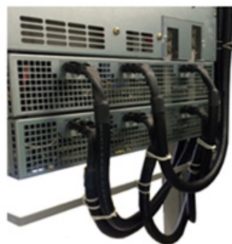
Figure 13: AC Cords Attached to Bracket with Lacing.
