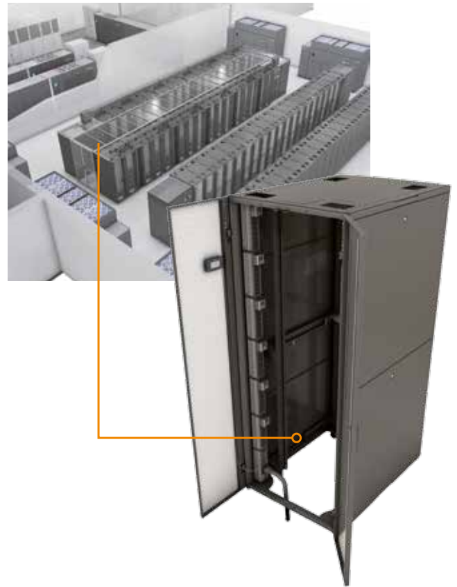
Figure 2. Located at the back of the rack toward the hot-aisle, rack PDUs can be exposed to temperatures exceeding 50 degrees Celsius.
