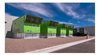
"The Liebert<sup>®</sup> air handlers allowed us to avoid building a central cooling plant, they matched our modular build design, which is important for both environmental and capital efficiency, and they enabled us to more tightly control the data center temperature and humidity."
