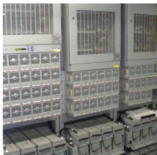
In the case of the Superdome, one provider leveraged a small room within the stadium as their headend. Three NetSure™ 721 DC power systems with two strings of batteries each and two battery racks with five more strings of batteries each were deployed to power the DAS network.
