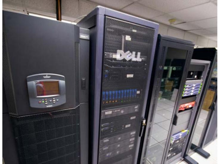
*By reconfiguring the data center’s existing IT infrastructure and replacing traditional perimeter cooling with a row-based solution, the A. James Clark School of Engineering at the University of Maryland doubled its capacity, increased the availability of critical systems and enhanced the data center’s overall efficiency.*
