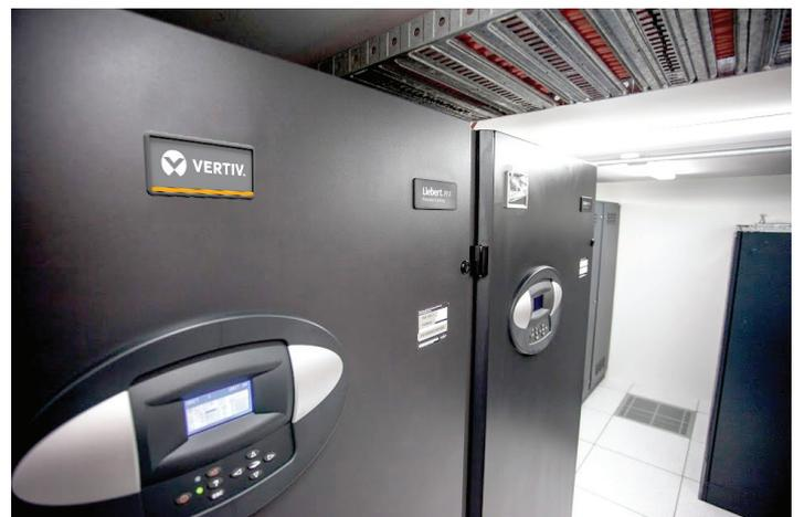
Liebert iCOM controls enabled Micron21 to see in real time the cooling capacity via a dedicated monitoring network. The system combination offers Micron21 complete redundancy, giving them the ability to switch between a completely closed chilled water system to an air and refrigerant cooled data centre. At the same time, the Liebert iCOM control, digital scroll technology and EC fans significantly contribute to achieving a low Power Usage Effectiveness (PUE).
