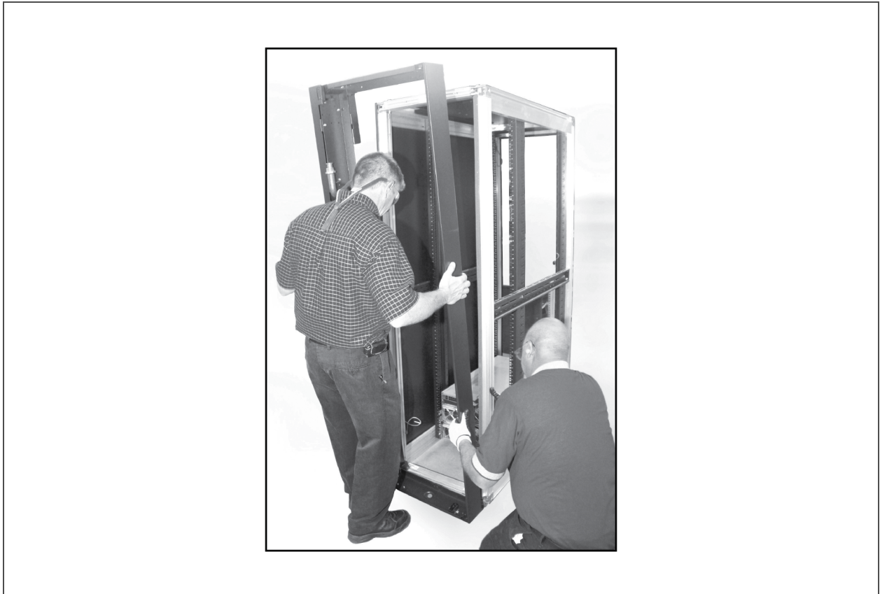
Figure 6.2 Align the DCD frame with the rack
